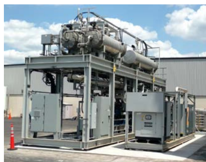
Figure 2: MTR 1MWe Polymeric Membrane System, installed and operational at a coal fired boiler
