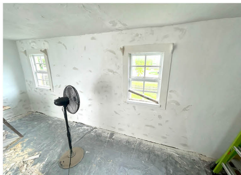
Kitchen wall repair @ RRTP
